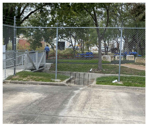
CONCRETE FLUME UNDER CHAINLINK FENCE
